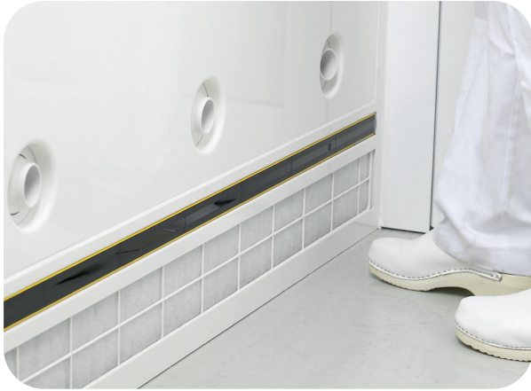
The lowest row of air nozzles is located close to the floor level for maximum efficiency.
